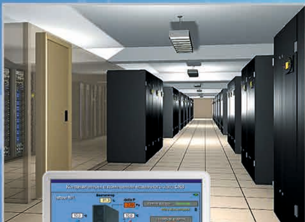
Control room of Parkoviy Data Center
