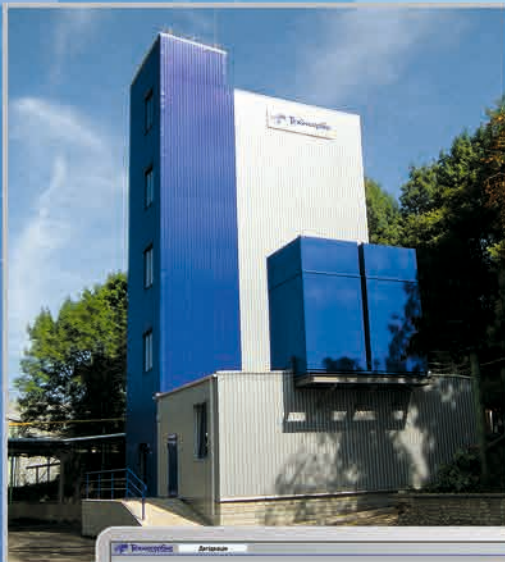
Ethanol dewatering station (fuel bioethanol production)
