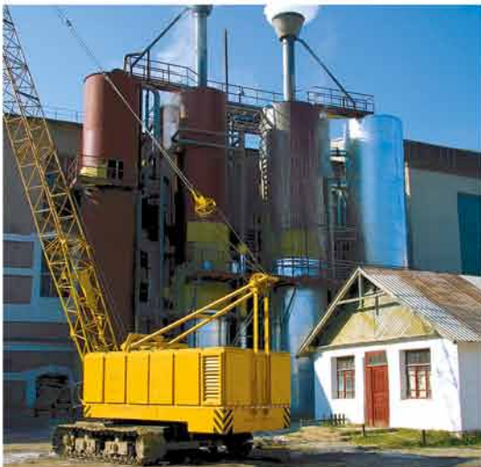
Insulation of Purification Station in Operation
